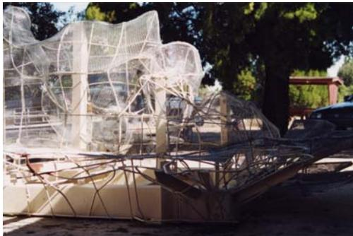
After the lathe was attached to the steel framework, a 1/4" cement scratch coat was applied to stiffen the cage.
